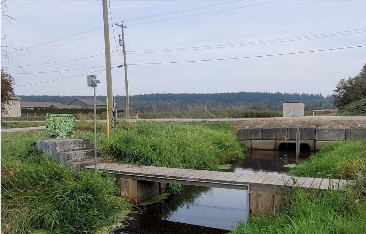
Figure 2: New monitoring site installed at Lorne Drain at 112 Street
