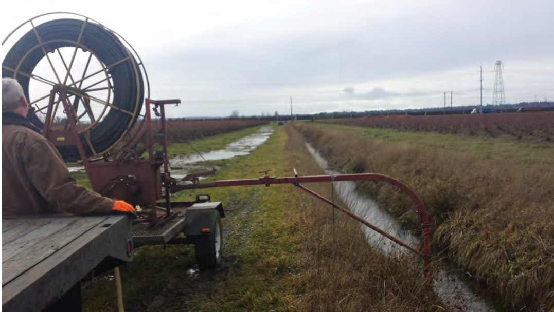
Figure 5 Contractor cleaning tile drains in a blueberry field
